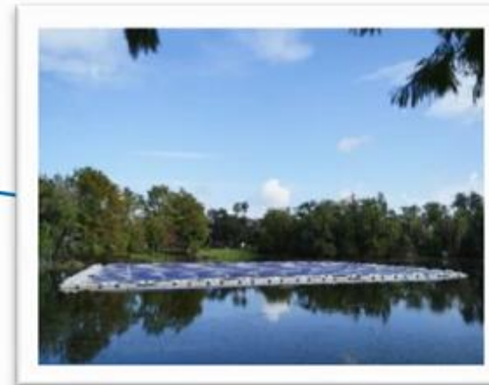
64kW Floating Solar Array
