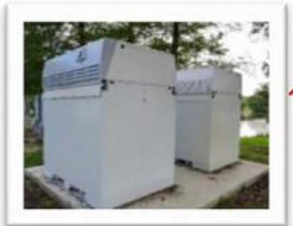
Two Vanadium Redox Flow Batteries
